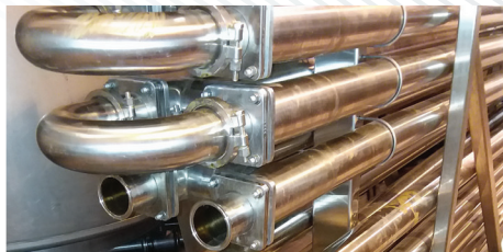
REPAIR BROKEN HEAT EXCHANGER
