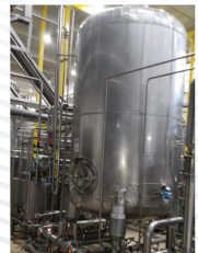
INSTALLATION OF NEW CARBON TANK
