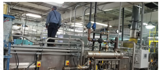
INSTALLATION AND CONNECTION OF NEW COOLING TUNNEL
